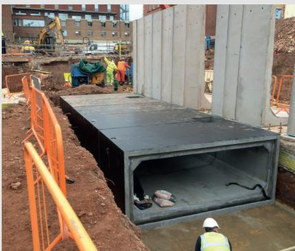
**Fabrication and erection of 550 tonnes of structural steelwork including a 15T truss. Installation of 300mm deep precast concrete flooring, Waycon lift shaft, culverts and a 20 ton Waycon stair core.**
